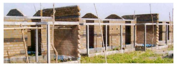
If the mountain soil indeed turns out to be unsuitable for pressing blocks, then it is worth to take a look at the other earth techniques. So the second recommendation is to explore the behavior of rammed earth for the rocky soils and adobe blocks for the finer soils.
